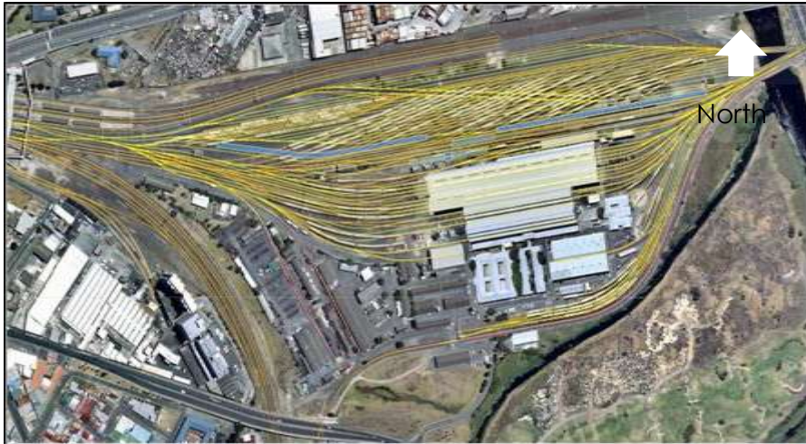
Figure 0-36: Salt River Train Depot Modernization *3
